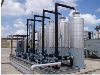
The Molecular Gate™ PSA unit
