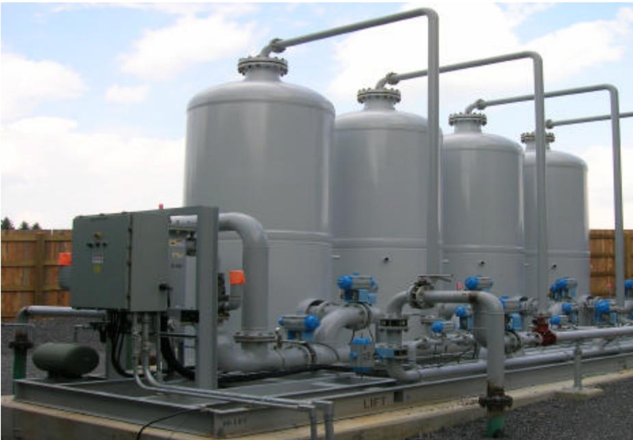
*Figure 3: Typical installation for a 2 - 5 MM SCFD Molecular Gate Unit*
