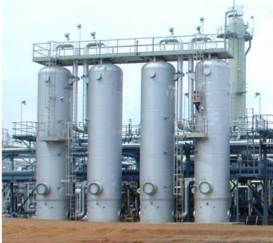
Figure 4 – A typical 4-vessel Sorbead Quick-Cycle Unit Oil-Drop Silica Gel
