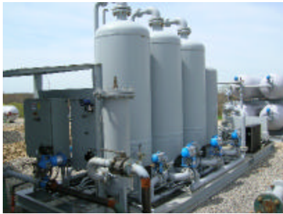
Typical Biogas Purification System
