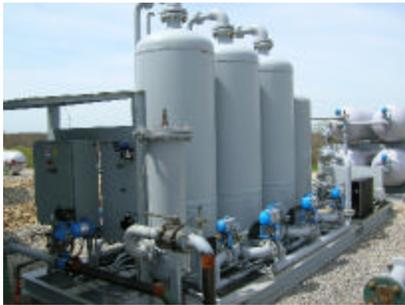
*Typical Biogas Purification System*
